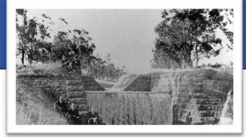
Drop on Aqueduct near Whittlesea (WHS Photo PD0785)
